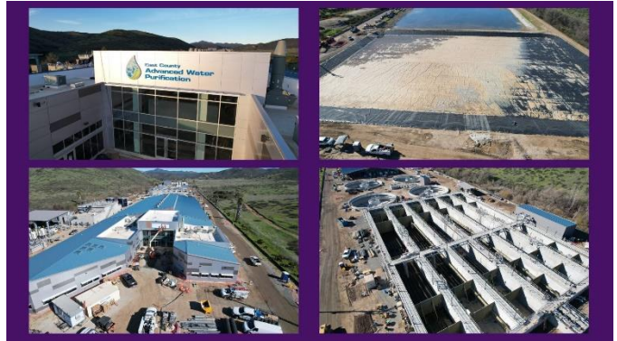
East County Advance Water Purification facility
