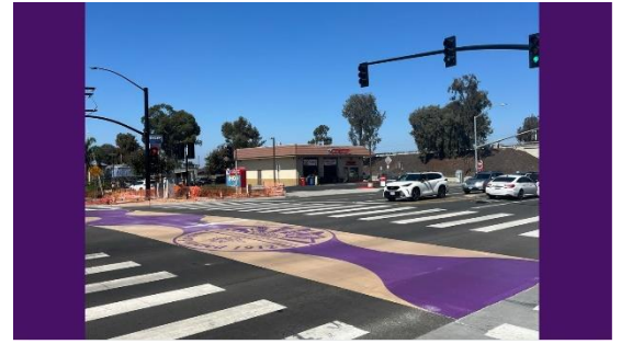
Intersection of Oakdale Avenue and N. Second Street
