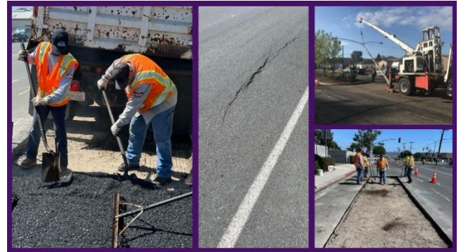
City Crews resurfacing roadways.
